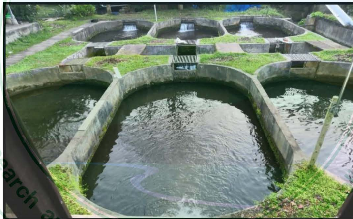
Figure 1: The 28 \text{ m}^3 experimental unit of concrete raceway
